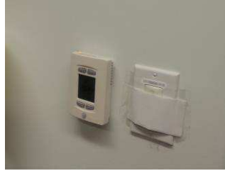
Figure 2: An example where the occupant taped over the motion detectors (taken from [44] credit: Sara Gilani).
