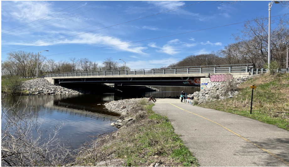
Fig. 7. Illustration of bridge in the test area
