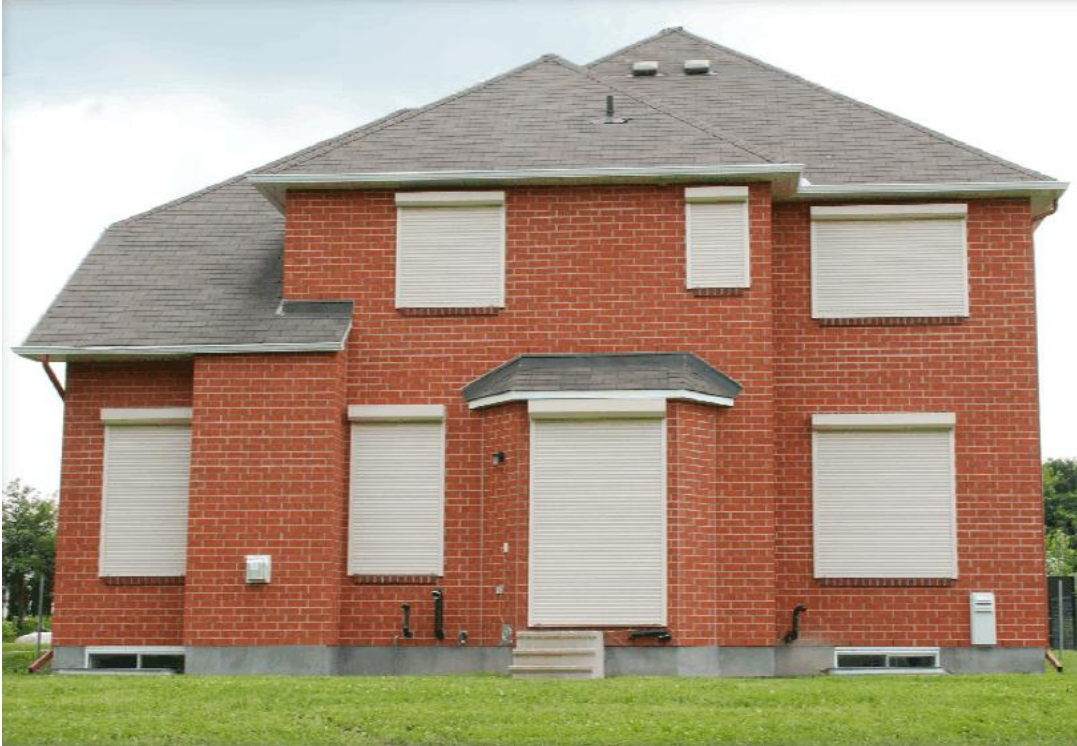
Figure 1. Rollshutters on the north side of a CCHT house.
