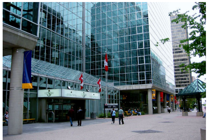
C.D. Howe Building in Ottawa
