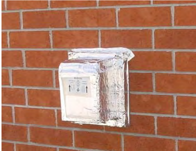
Figure 5 - Sealed fireplace vent during Benchmarking
