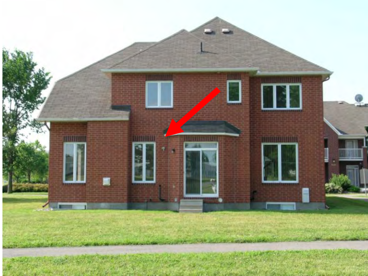
Figure 7 – North face of the CCHT Reference House, showing the location of the outdoor temperature sensor.
