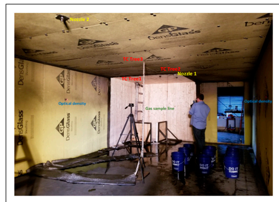
Figure 2. Test compartment and instrumentation.
