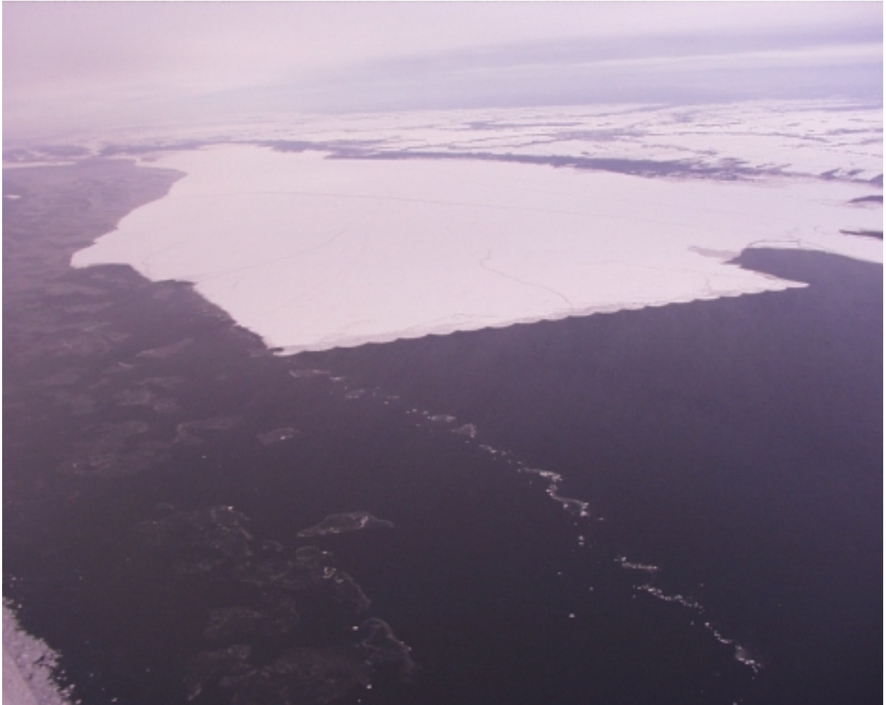
Figure 9.3 The 2.5 km wide Yamachiche boom viewed from the N-E towards the S-O. At the bottom of the image is the boom. On the viewer's right is the north shore. On the left is the navigation channel. The ice cover is partially retained by artificial islands (too small to see). Further upstream, the cover has a triangular shape because it is unconfined to its right (left side of image).
