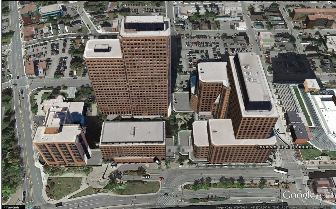
Figure 1: Les Terrasses de la Chaudière Complex, showing Block 100 (right), Block 200 (centre back), Block 300 (centre front), and the hotel (left, not part of project). (Picture from Google Earth)
