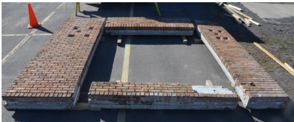
Figure 20 – As received LTDLC wall panel on the ground
