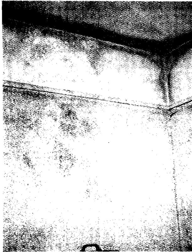
Condensation traces in the room of a ground floor apartment at the gable end on cold spots produced by the corners of the floors and the external walls
