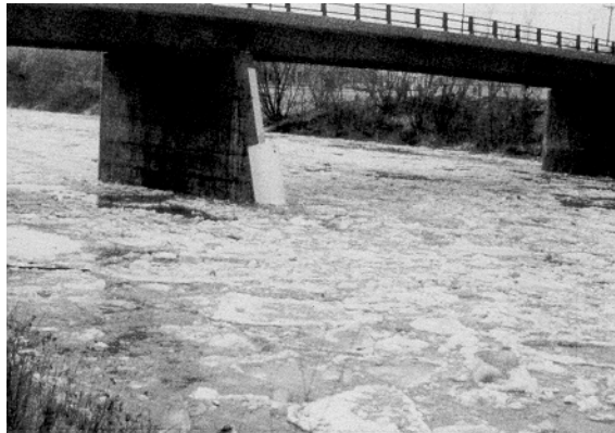
Figure 1 Bridge pier in the White River, Vermont (from Zabilansky, 1996)
