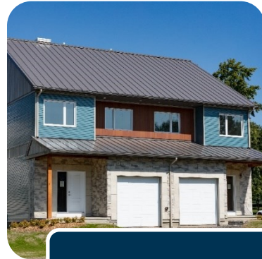
Resilient Residential Retrofit
