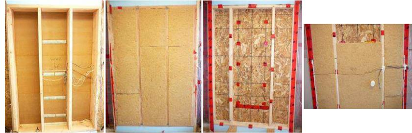
**Figure 7. Wall 2 (PH) - (i) Stud wall wood frame with diffusion board, (ii) wood fiber insulation in stud cavities, (iii) OSB smart vapour retarder (iv) interior wood fiber insulation**
