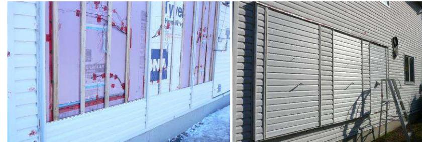
**Figure 9. Installation of W1, W2, & W3 in FEWF showing (i) exterior layers under air cavity, furring strips & (ii) exterior cladding (vinyl siding)**
