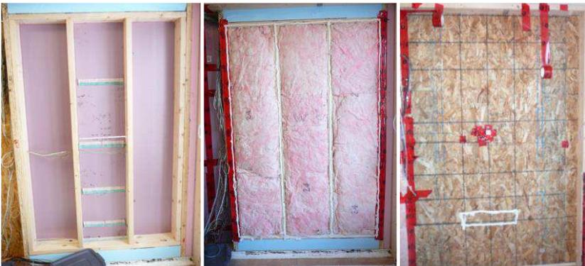
**Figure 8. W3 (OSB) – (i) Stud wall wood frame with external XPS board, (ii) GF batt insulation in stud cavities, (iii) OSB smart vapour retarder**
