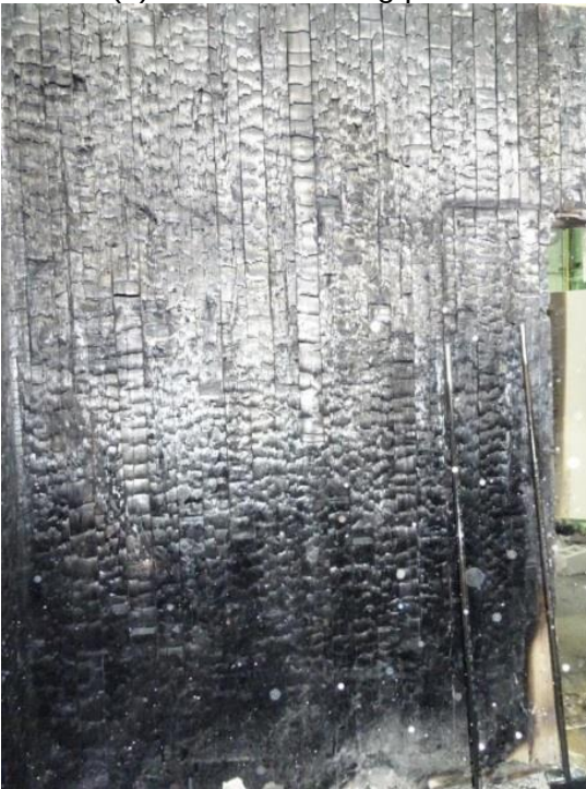
(c) CLT panel from Wall C
