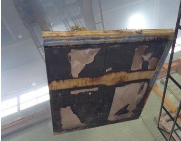
(a) lifted CLT ceiling panel
