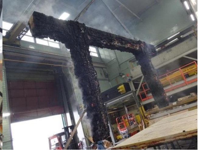
(b) lifted Glulam beam and columns
