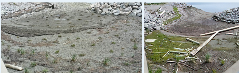
Figure 11.7. Salt Marsh Vegetation Establishment on Leeward Side of the Barrier Islands
