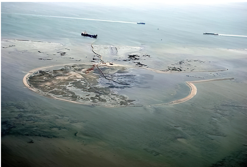
Figure 11.12. Construction at the Galgeplaat (the Netherlands)
