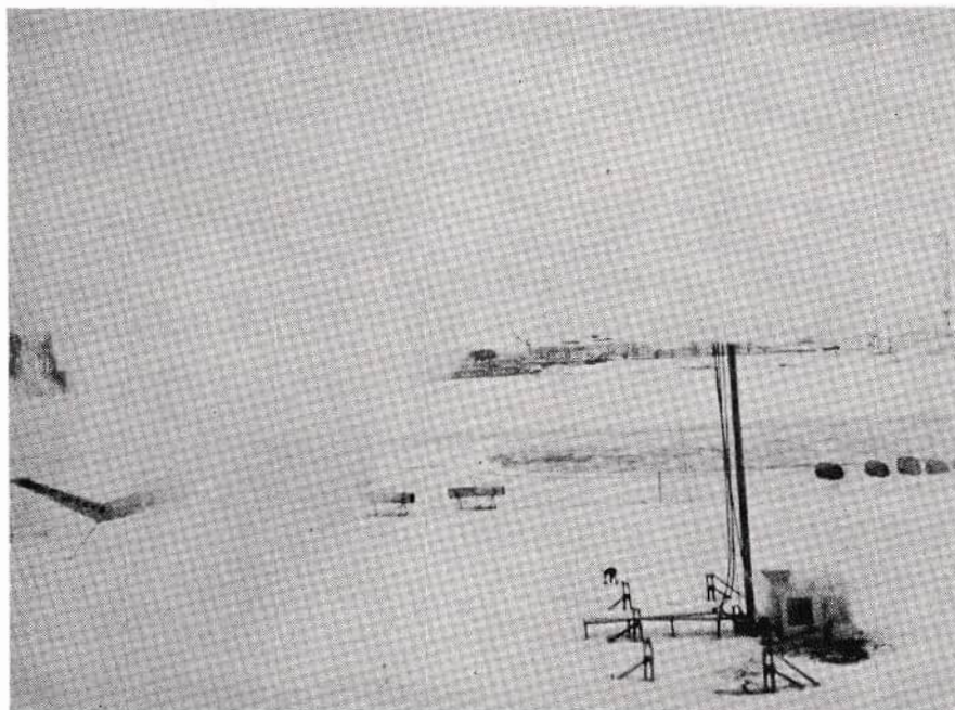
(b) GENERAL VIEW FROM THE AIR OF HUT INSTALLATION
