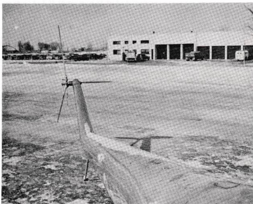
EXTENT OF ICE ON TAIL CONE AT -16^{\circ}\text{C}
