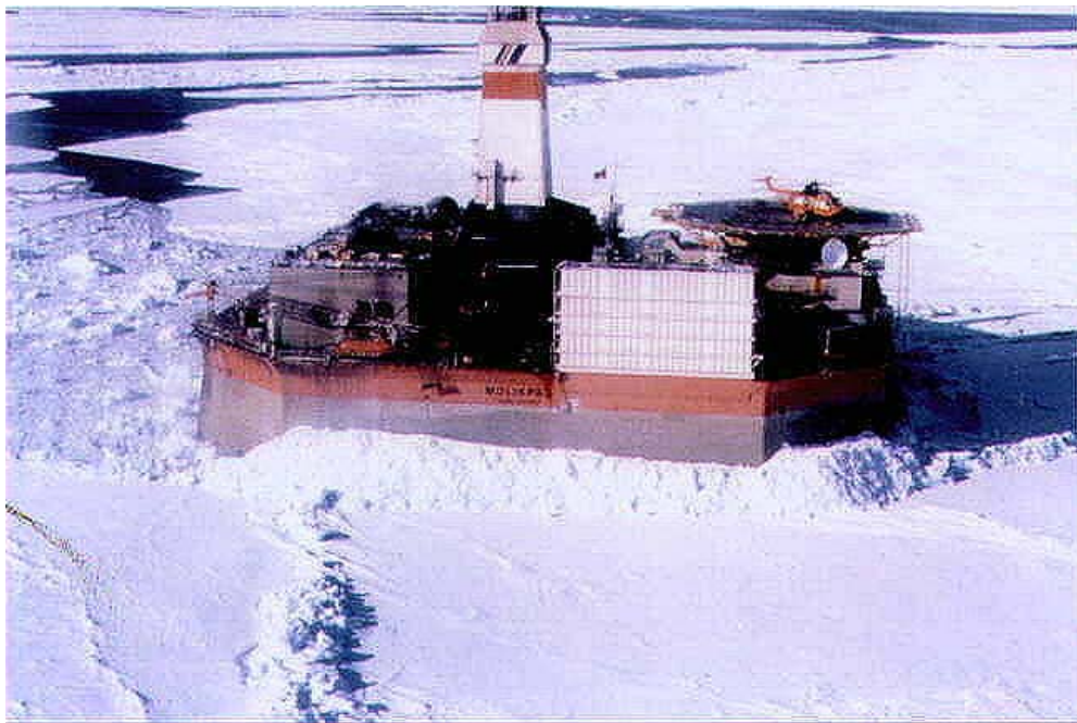
Figure 1-1 The Molikpaq at location with ice crushing against two sides
